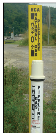
5. HCA marker and cathodic protection test station
