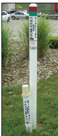
2. Linemarkers and cathodic protection test station
